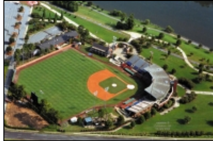
Aerial view of Historic Golden Park in Columbus, Georgia.
